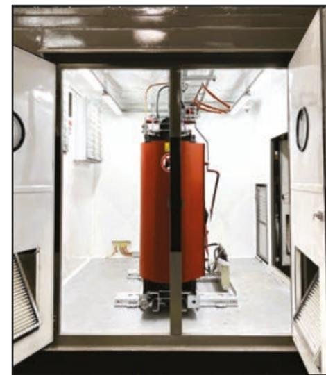
data centre project in the Netherlands, where it is supplying three 22,5 MVA, 50 kV/13.8 kV dry-type transformers being used in the intake substation, demonstrating the company's expertise in delivering customised solutions to meet unique project requirements.
